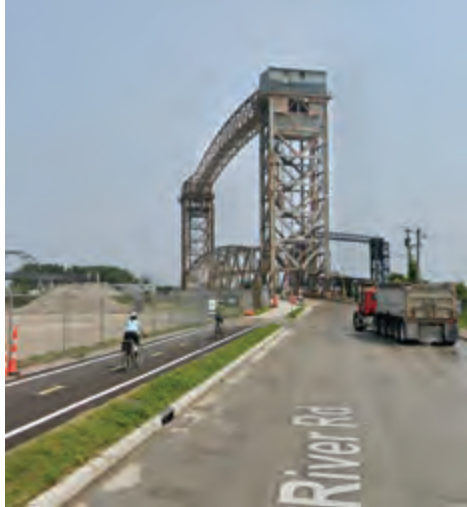
The Whiskey Island connector connects the Centennial Lake Link Trail, the Towpath, and Edgewater Park to Whiskey Island.
