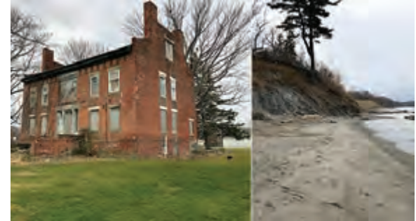
Parmly Mansion and the Perry Township shoreline by KS Associates.
