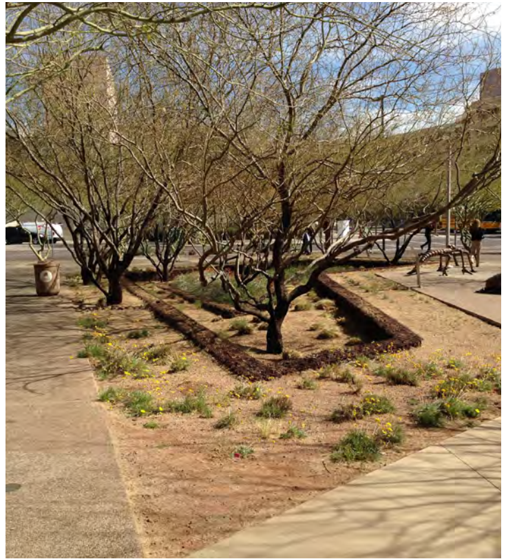
A bioretention cell in downtown Phoenix, AZ. These systems can be used in many different climates, but sensitivity to local conditions and native plants is necessary. Photo credit: John Rozum
