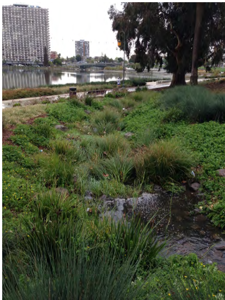
Bioswale used for stormwater runoff near downtown Oakland, CA. Photo credit: John Rozum
