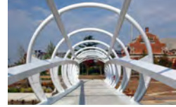
NEW PEDESTRIAN BRIDGE
