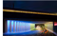
LIGHTING AT HIGHWAY CROSSINGS
